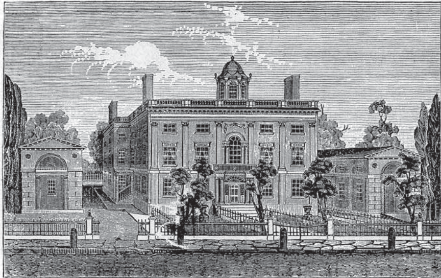
DERBY MANSION, BUILT IN 1799 ON PRESENT SITE OF MARKET HOUSE, SALEM. COST $80,000.
