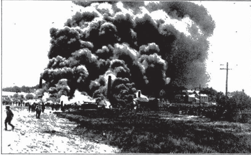
Fire at Works of Salem & So. Danvers Oil Co. June 14, 1887.
