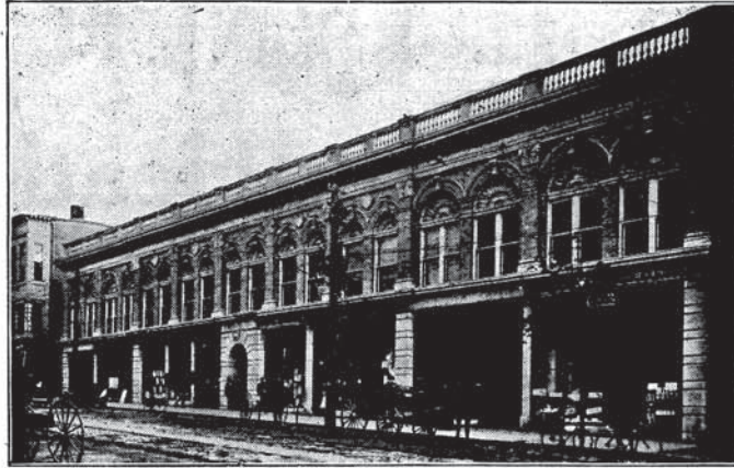
O' SHEA BUILDING, PEABODY, Built by
